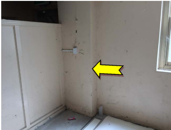
Photo 9. Interior, throughout, walls – suspected lead-containing cream upper paint system.
