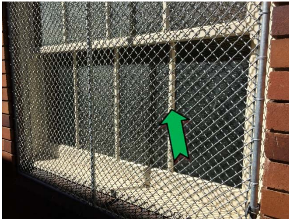
Photo 3. Exterior, throughout, window frames – non asbestos-containing window caulking.
