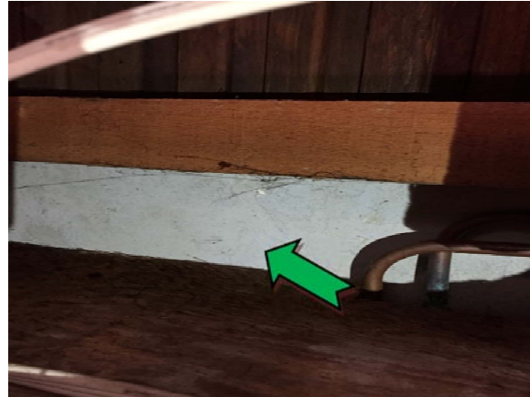
Photo 2. Interior, basement level, multi-function hall, ceiling – non asbestos-containing fibre cement sheeting.
