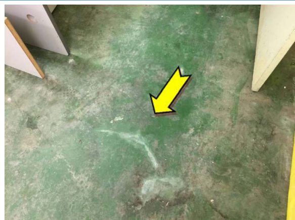
Photo 12. Interior, basement, fire-proof storage room, bathrooms & corridor, floor – suspected lead-containing green upper paint system.
